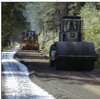
Figure 3. Compacting after in-place processing
