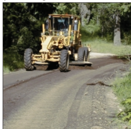
Figure 4. Grading after in-place processing
